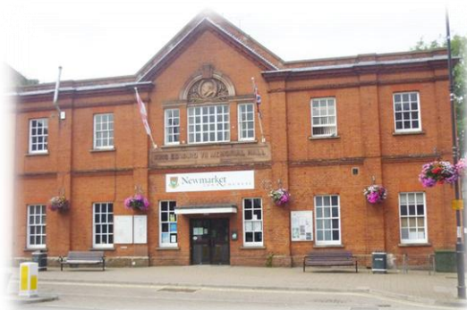
King Edward Memorial Hall, Newmarket Copyright © Julian Osley
